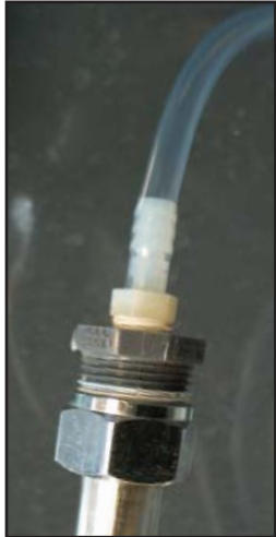
J. Hose barb adapter & 1/4" hose used to make temporary connection from softener outlet to drain.
